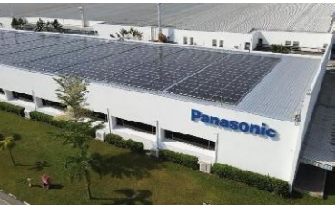
Photovoltaic power generation systems at Malaysia Site
